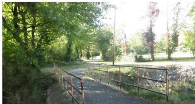
Greenway Bikeway: Existing bridge railings do not meet current standards and should be upgraded.
