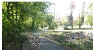
Greenway Bikeway: Existing bridge railings do not meet current standards and should be upgraded.
