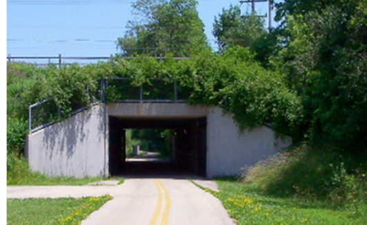
Typical Box Culvert Pedestrian Tunnel
