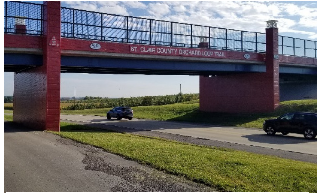
Steel Beam Bridge along MetroBikeLink, with formliner finish and concrete staining.
