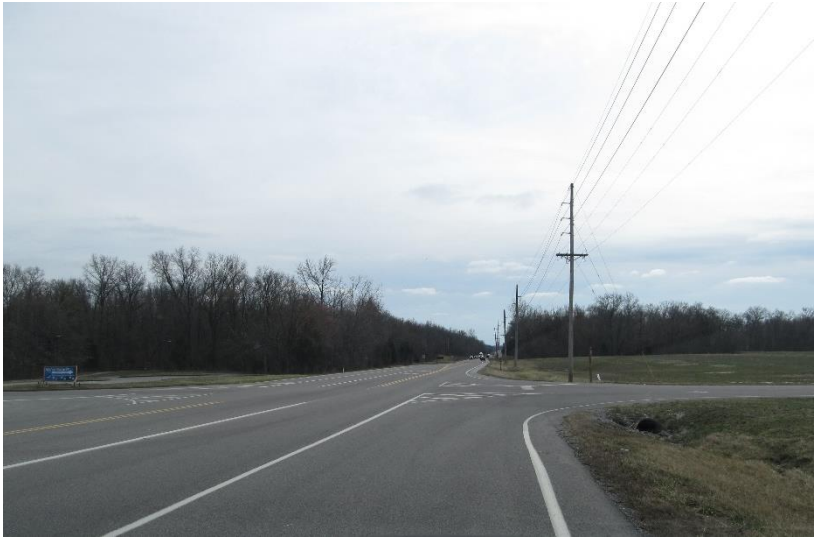
Intersection of IL 148 and Pigeon Creek Road
