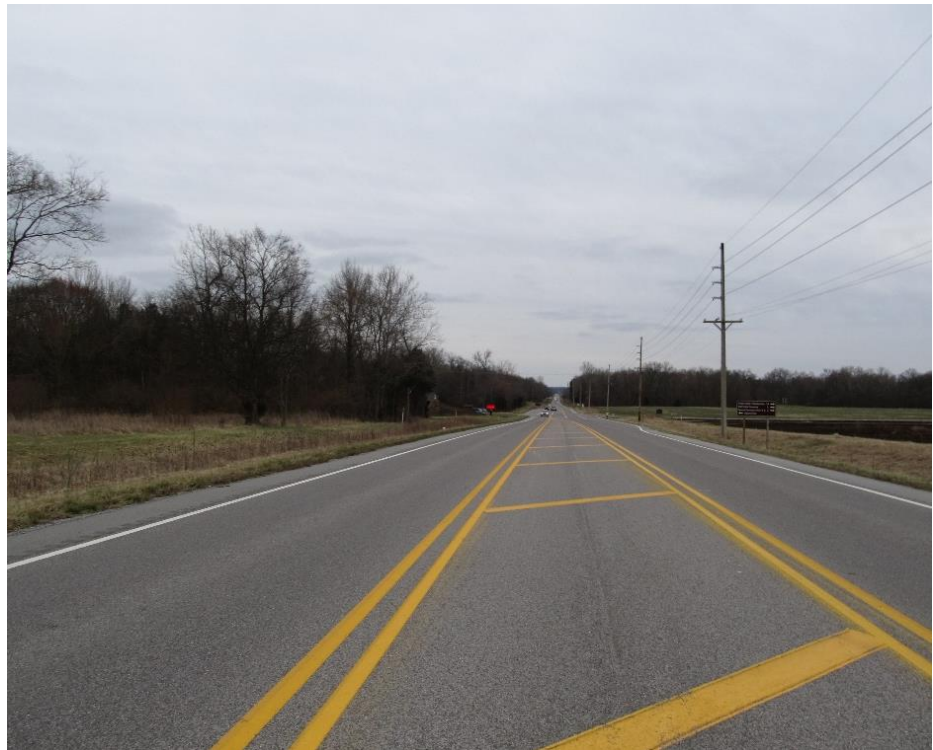
IL 148 - Looking South Approaching turns lanes at Pigeon Creek Road
