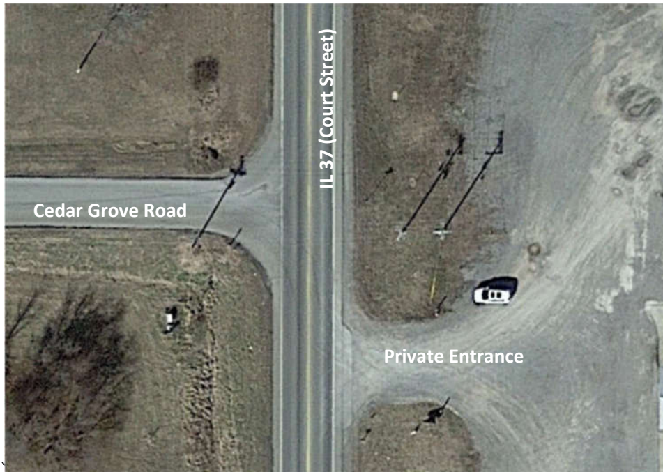
Figure 3: The Intersection of Illinois 37 and Cedar Grove Road
