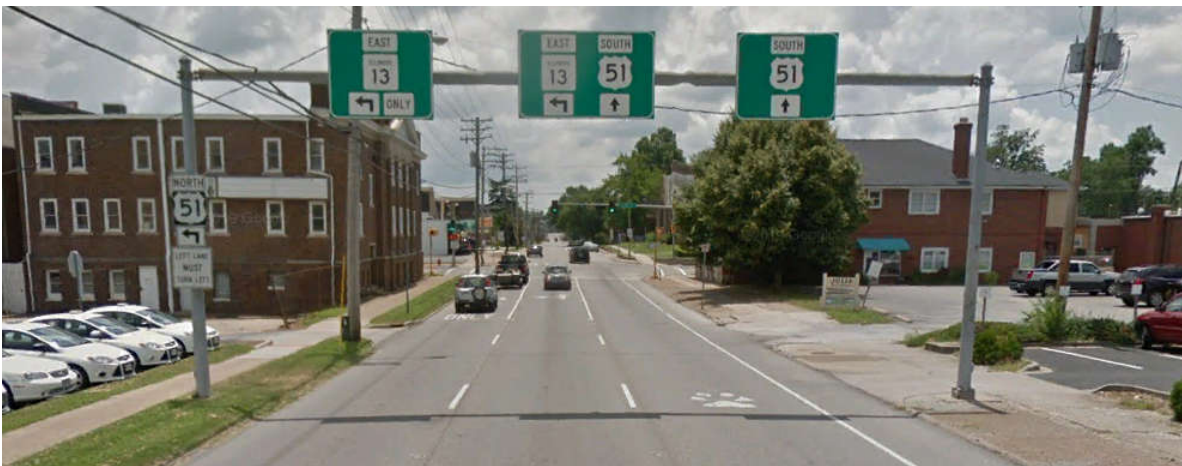
Figure 4: Southbound on University Avenue North of the Intersection (Looking South)
