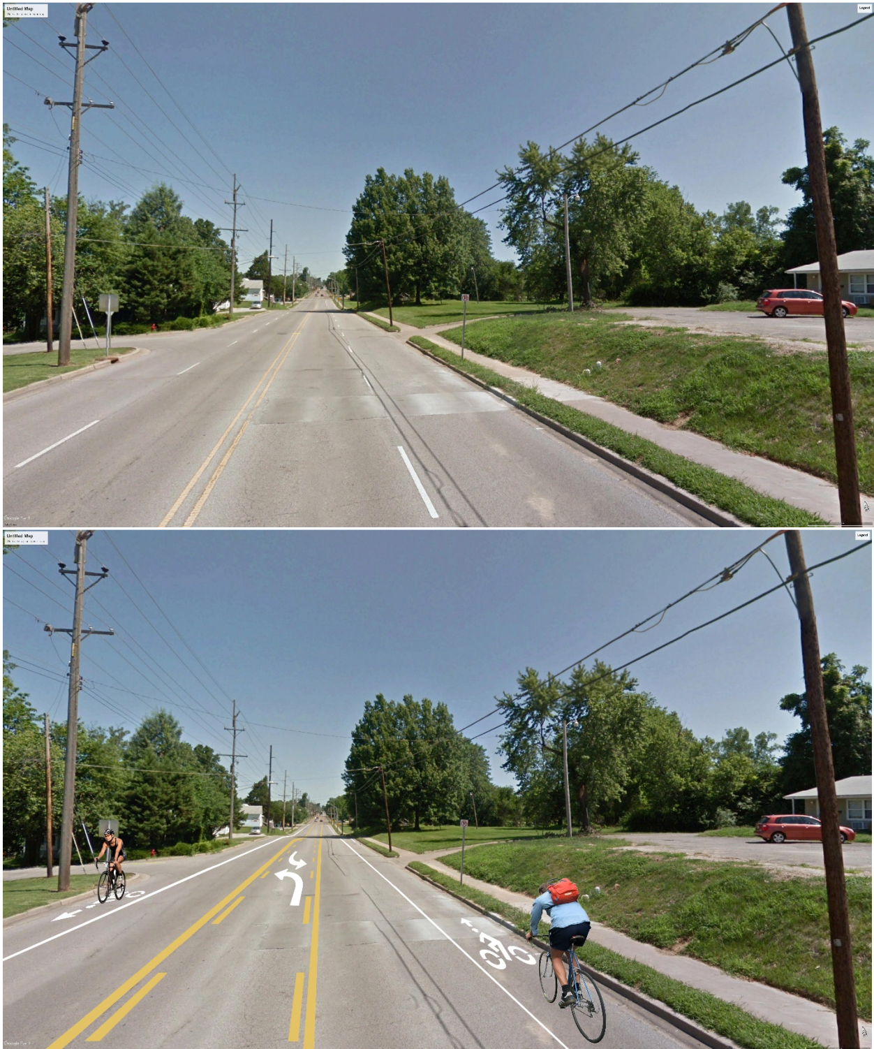
Figure 21. Before (top) and After (bottom) Wall Street Road-Diet Conversion
