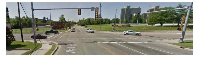
The alignment of the west leg is comprised of an S-curve (see **Figure 2**). The existing EB lane configuration at the intersection drops the inside through lane directly into the EBLT lane.
