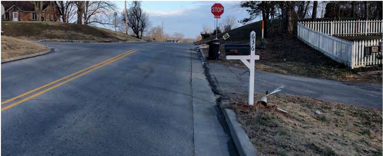
E. Pleasant Hill Road is a curbed roadway having an overall width of 31 feet from back to back of curb. A double yellow centerline is the primary pavement marking with the exception of the westbound approach to Wall Street -- a second westbound lane and a painted median is added to shadow an opposing left-turn lane (**Photo 3**). The eastbound approach of the E. Pleasant Hill and Wall Street intersection has an exclusive left-turn lane and a through lane.
