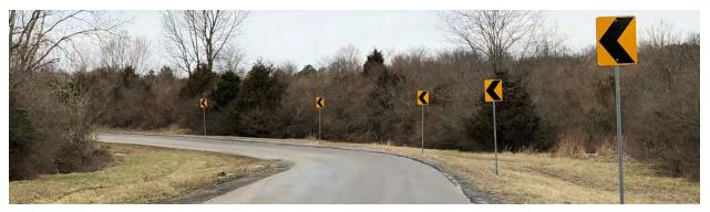
**Photo 11** shows chevrons on Curve #3 from the perspective of Curve #2 on northbound Crenshaw Road. Additional chevrons along the horizontal/vertical curve of Curve #2 (red arrow) are recommended.
