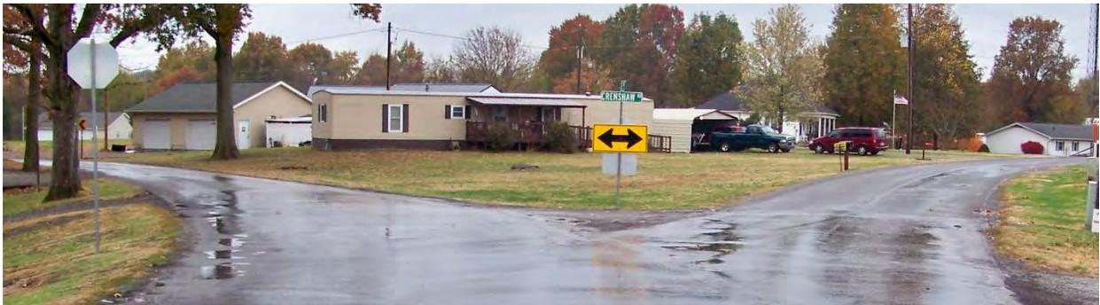
The Skyline Road and Crenshaw Road intersection has 3-legs and is configured as a T-intersection. The stem of the T-intersection (Skyline Road) is stop controlled whereas the Crenshaw Road approaches have right of way. The posted speed limit on Skyline Road is 50 MPH.
