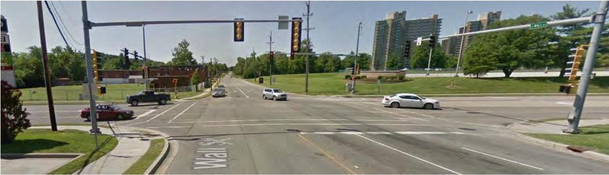
The alignment of the west leg is comprised of an S-curve (see **Figure 2**). The existing EB lane configuration at the intersection drops the inside through lane directly into the EBLT lane.
