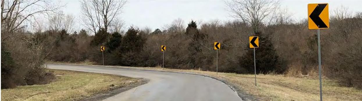
**Photo 11** shows chevrons on Curve #3 from the perspective of Curve #2 on northbound Crenshaw Road. **Additional chevrons along the horizontal/vertical curve of Curve #2 (red arrow)** are recommended.
