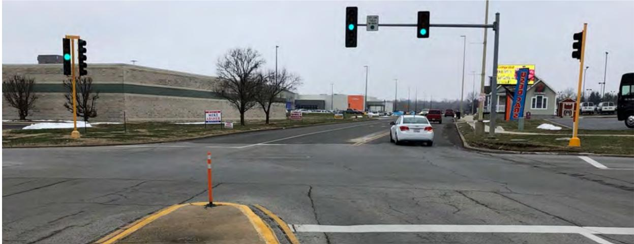
**Photo 3** shows rutting in the NE quadrant of the intersection. The curb radii are equal to 25 feet on all quadrants of the intersection. Photo 3 also shows the position of the side street stop lines being less than 10 feet from the edge of the cross street.
