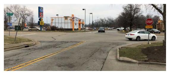
• Westbound Frontage Road. Two lane approach with an auxiliary left turn lane. The approach is stop-controller. Note stop sign condition on Photo 2. A supplemental warning sign exists under the Stop Sign which reads "Traffic From Left Does Not Stop." Pavement markings were recently upgraded. Single line centerline exists on the westbound approach. The aerial view of Figure 1 shows the centerline pavement markings were worn/not existent.
