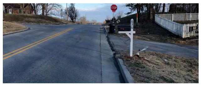
E. Pleasant Hill Road is a curbed roadway having an overall width of 31 feet from back to back of curb. A double yellow centerline is the primary pavement marking with the exception of the westbound approach to Wall Street -- a second westbound lane and a painted median is added to shadow an opposing left-turn lane (**Photo 3**). The eastbound approach of the E. Pleasant Hill and Wall Street intersection has an exclusive left-turn lane and a through lane.
