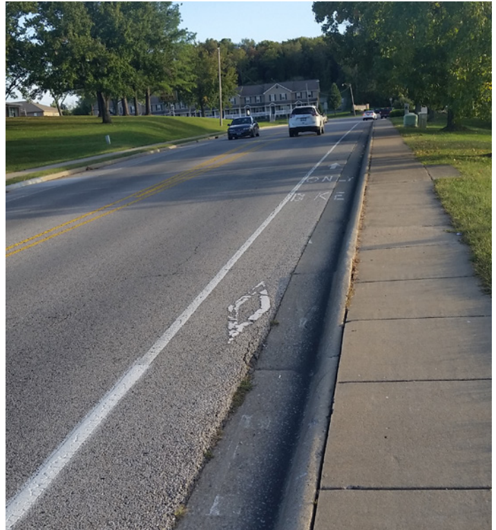
Lewis Lane is an example of a street where the existing striping does not meet the standard for a “bike lane” and there is not enough within the street to restripe for a full bike lane. In this situation, the striped area should be referred to as an “Urban Shoulder”. (Note: this existing urban shoulder incorrectly has bike lane markings. Bike lane markings should only be used on “official” bike lanes.
