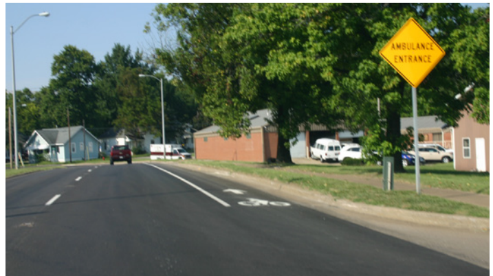
Existing bike lane along University Avenue.
