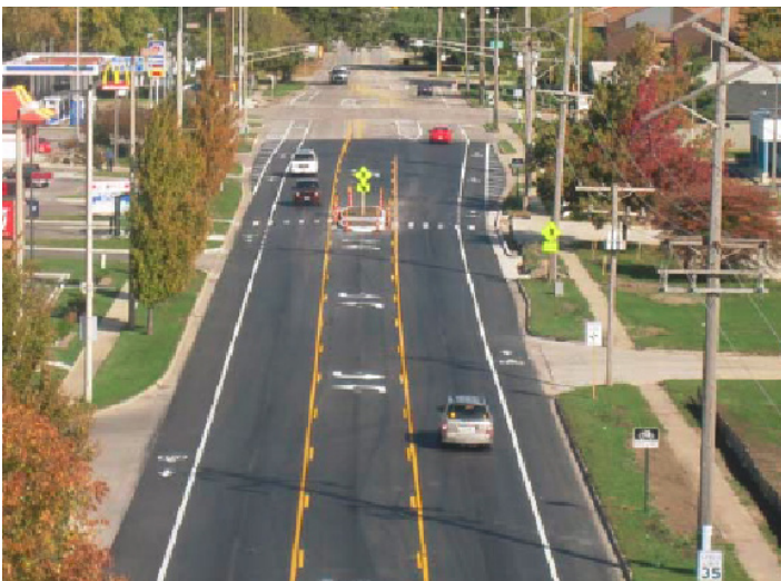
Example of a road diet in Urbana. This road was previously four lanes.
