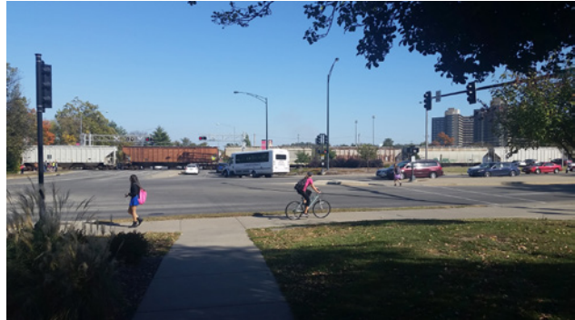
The intersection at Grand Avenue and Illinois Avenue is a key gateway for bicyclists and pedestrians to campus.
