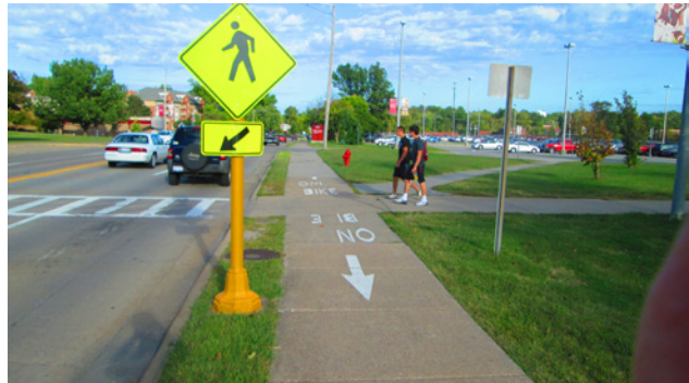
Replace existing continuous flash beacon with RRFB. Widen existing sidewalk to 10' sidepath.
